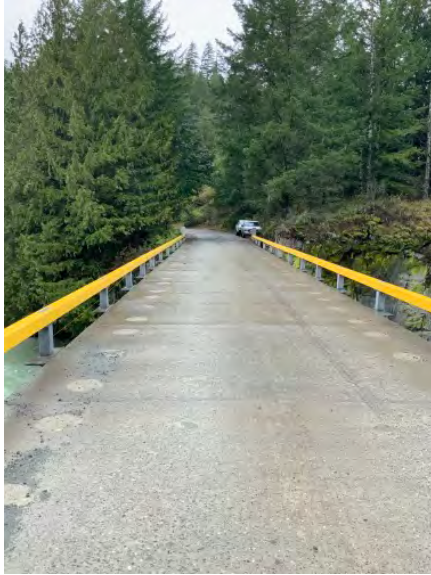
Approach from Right Bank when facing downstream
