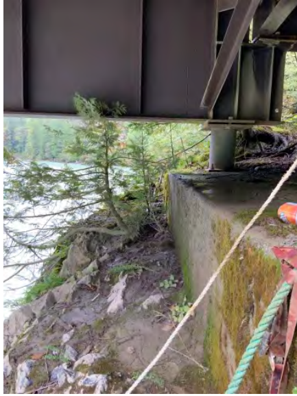
Left Bank Abutment when facing downstream
