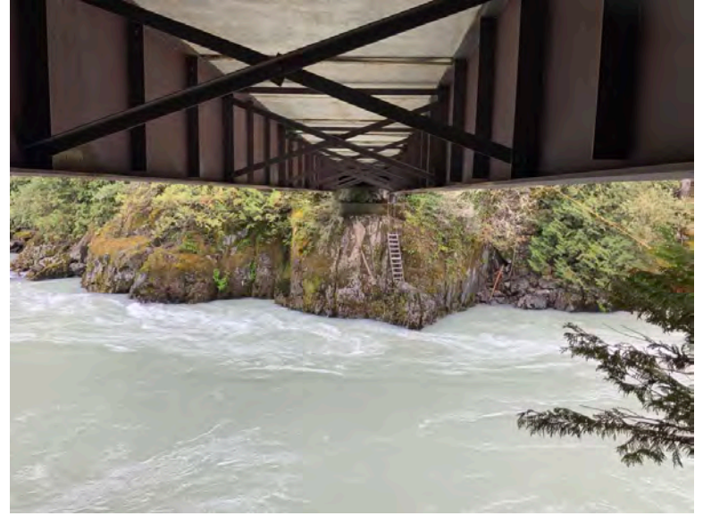
Left Bank Abutment when facing downstream
