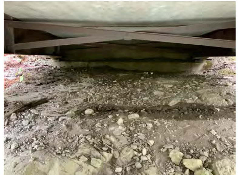
Left Bank Abutment when facing downstream on jump span left end
