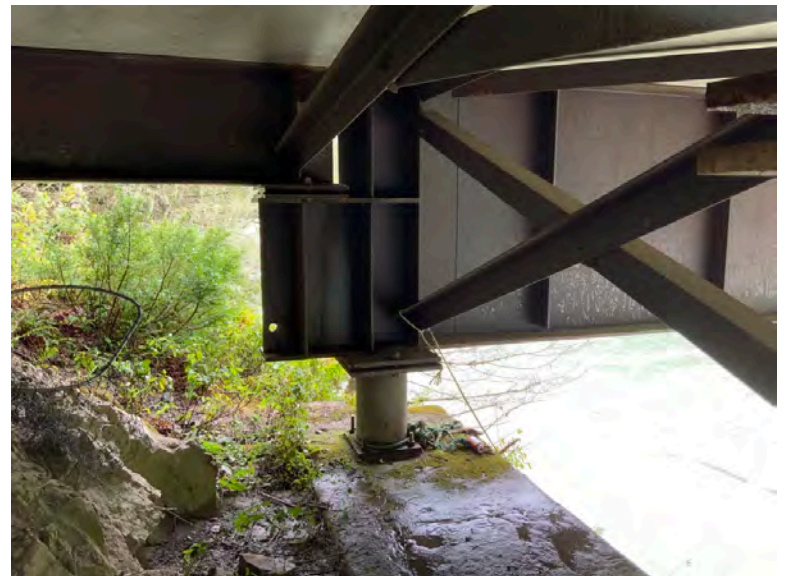
Left Bank Abutment when facing downstream
